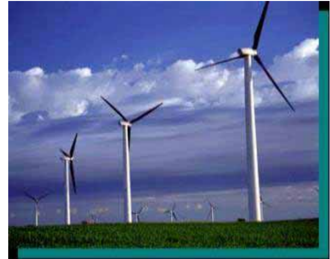
NSP 107 MW Lake Benton wind farm 4 cents/kWh (unsubsidized)
